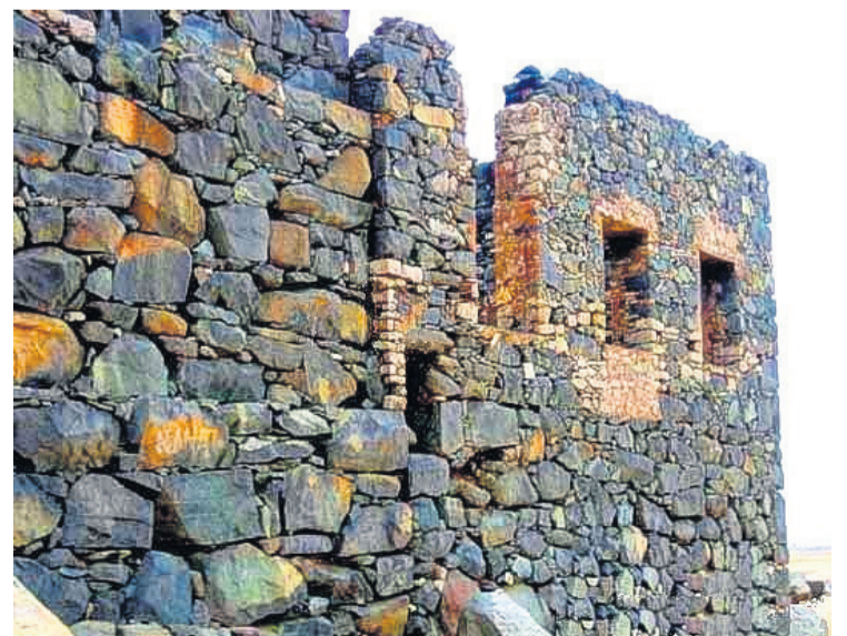
Pic. 3, the implementation of local stones as construction material at Bushiribana, Paradera .
